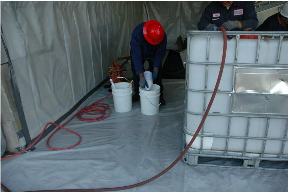
Photo #8: Preparing cleaning solutions. Note tank for capturing spent water
