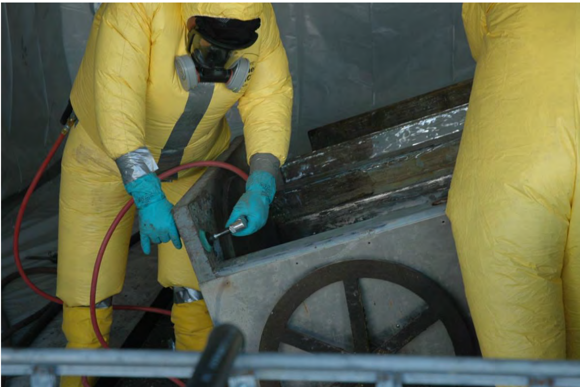
Photo #16: Using an air operated plastic brush to remove debris
