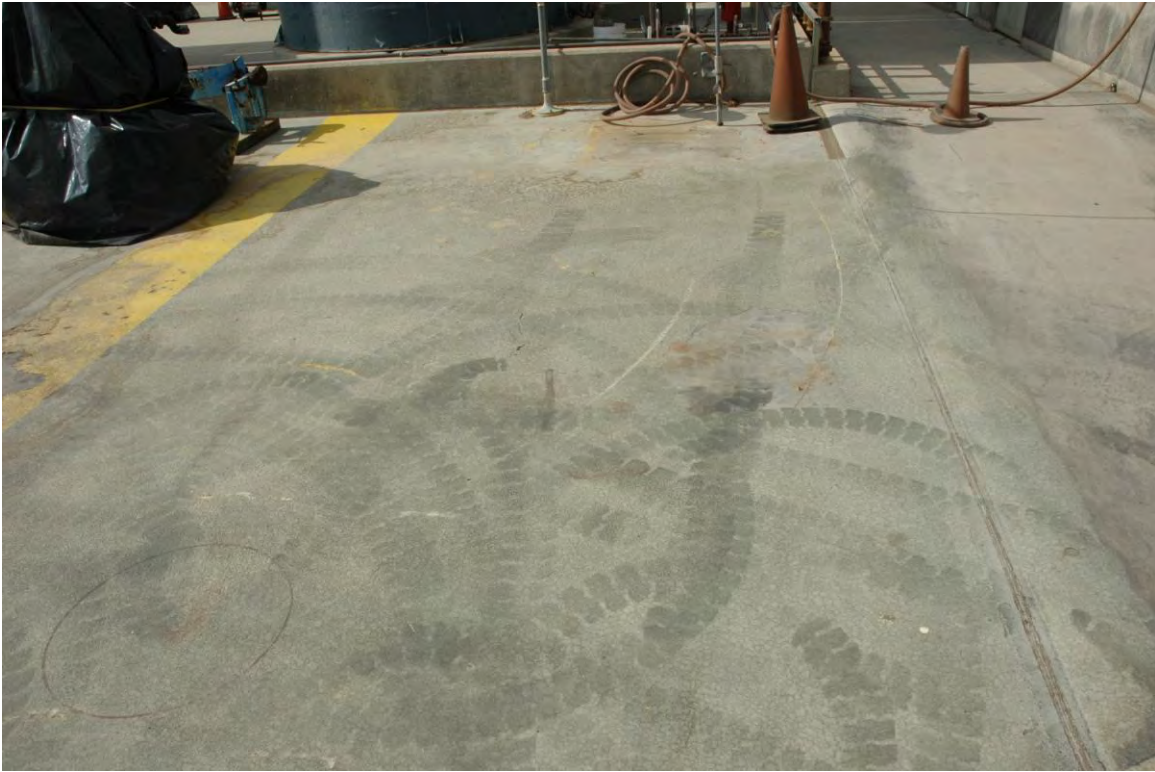
Photo #25: Pad where machine was removed – No visible cracks
