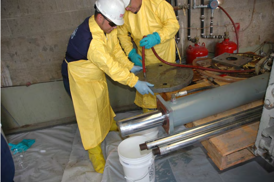
Photo #17: Rinsing of plunger- note plunger was rotated in 90 degree increments until all surfaces were rinsed
