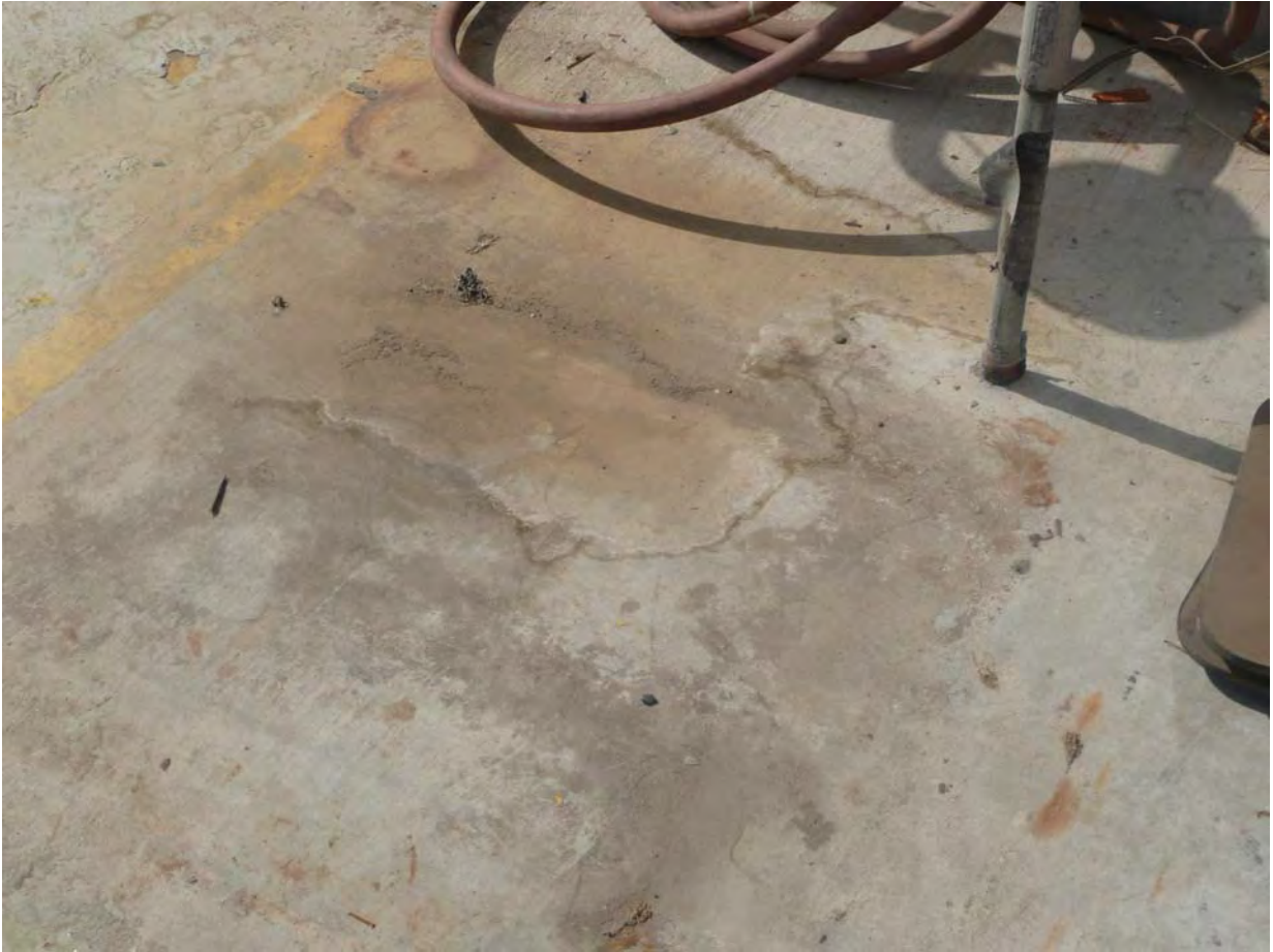
Photo # 26: Close up of containment pad where WCU was removed. Visible chipping in containment coating can be seen.
