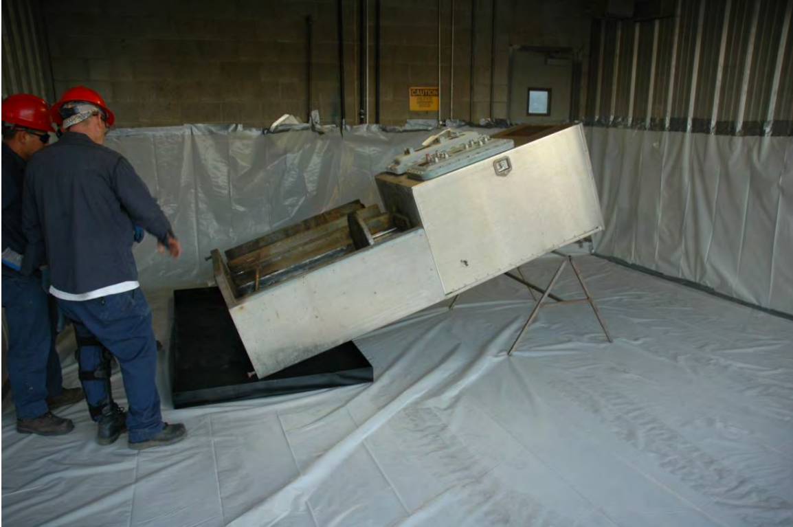
Photo #7: Unit placed in cleaning area – on angle to permit drainage
