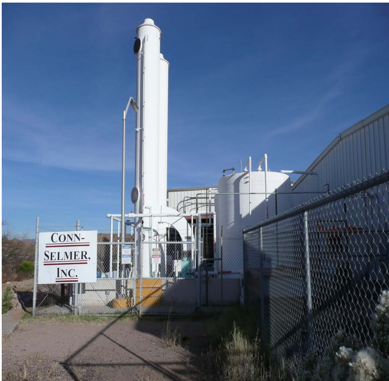
Figure 4 - Photograph of the Groundwater Remediation System
