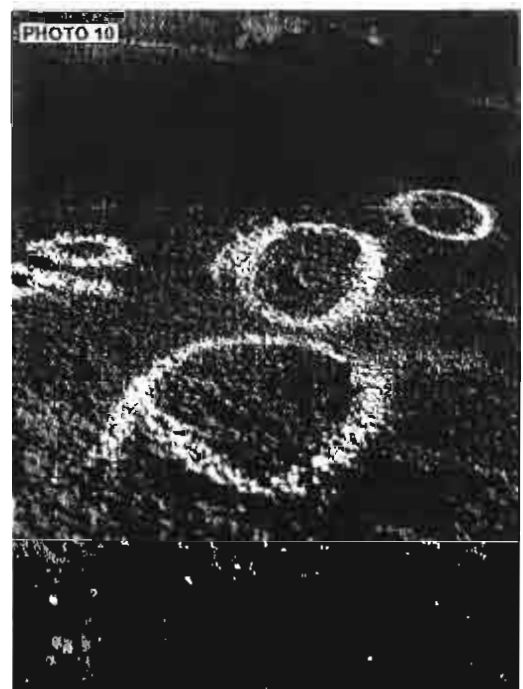
INTERIOR, TANK BOTTOM; VIEW SHOWING CORROSION
