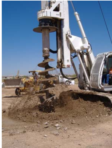
IA-11 Injection Well Installation
