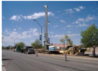
IA-12 Injection Well Installation
