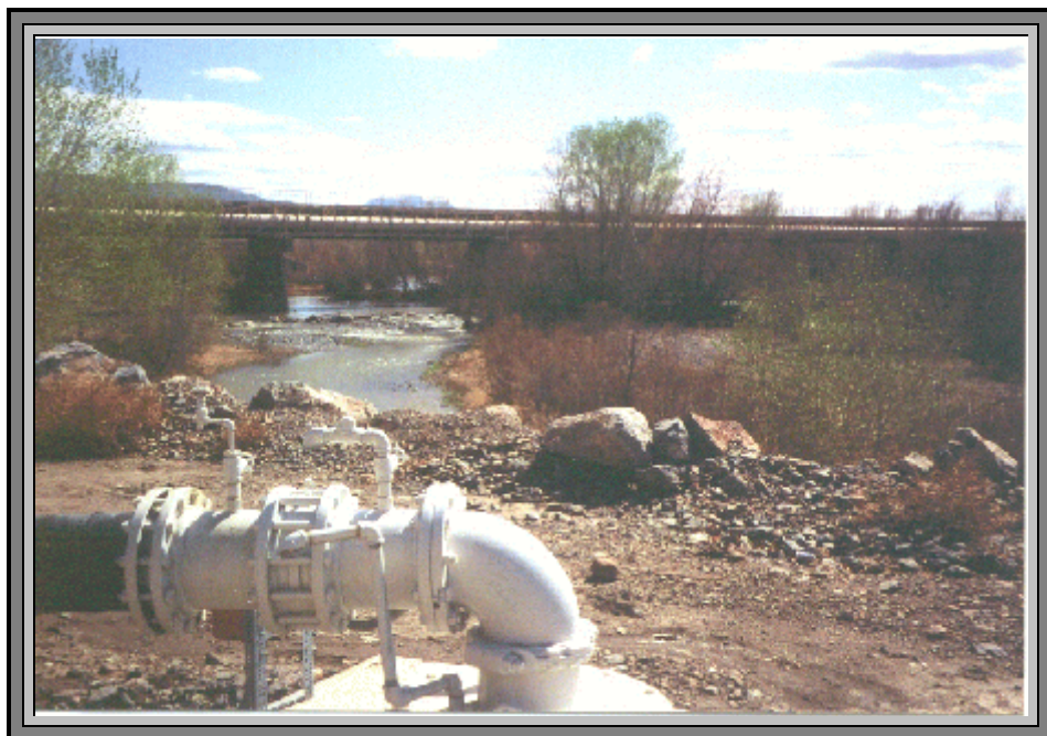
Figure 29. The highest sulfate concentrations usually occur in wells withdrawing water from the floodplain aquifer, particularly those between the towns of Mammoth and Kearny. One such well that exceeds the 250 mg/l Secondary MCL is pictured above, which supplies water to ASARCO's milling activities near the town of Hayden. The influence of surface water recharge from the Gila River to nearby shallow wells is evident in this photograph.
