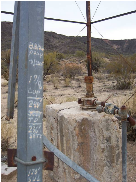
Figure 7 – This isn't graffiti left on a stanchion of Broken Windmill (BWM-58) but rather informative hydrologic notes left when Balow Pump last serviced the well. The well is 244 feet in total depth, the pump is set at 236 feet, the static water level is 170 feet, and the cup size for the leathers is 1 7/8 inches.
