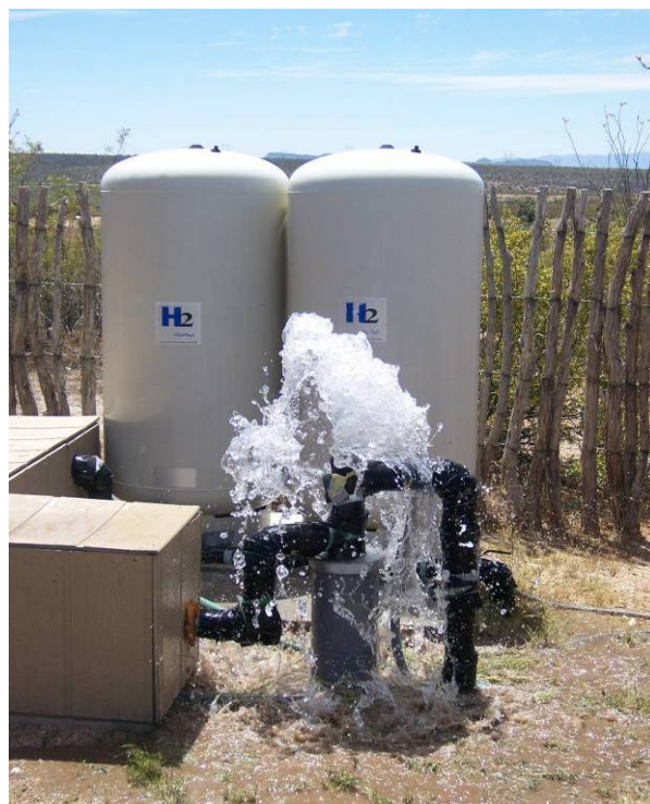
Figure 10 – A domestic well located near Date Creek is being purged prior to sampling. The sample (BWM-104) collected from the well met all water quality standards.
