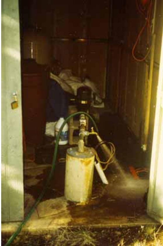
Figure 2. This 400-foot domestic well (HUA-1) shows the preferred sampling location of a faucet located near the wellhead.
