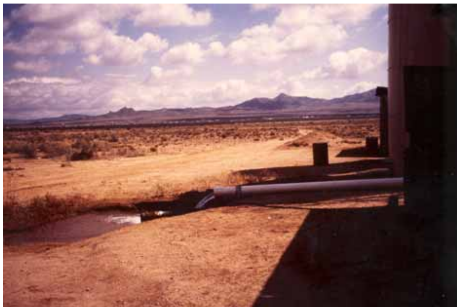
Figure 7. Some wells in the Hualapai Valley basin are capable of producing upwards of 1,000 gallons per minute, such as this irrigation well off Route 66 between Kingman and Hackberry. This well was 1,059 feet deep and the sample (HUA-27) met all health-based water quality standards.
