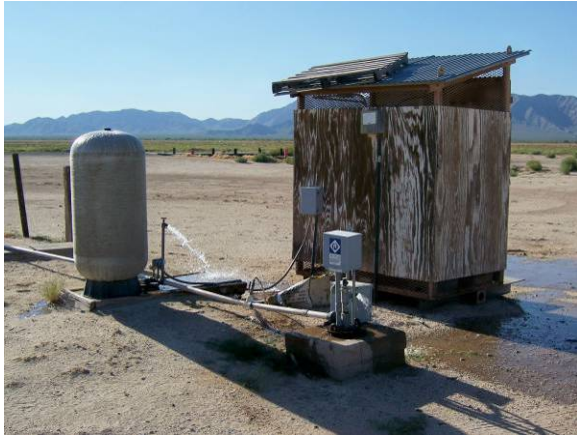
Figure 7 – This 970-foot, domestic well tapping the Western Regional aquifer met all water quality standards; only water quality guidelines for pH-field and fluoride were exceeded.
