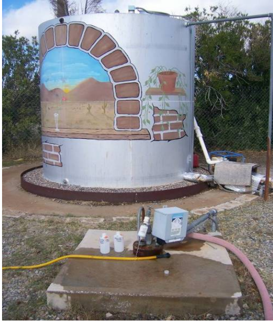
Figure 11 – This 500-foot well provides water to irrigate the grounds of a trailer park just northeast of Salome. Unfortunately, due to the absence at this location of the Lake-bed Unit, the Regional aquifer merges with the poor quality water in the Perched aquifer to form the Mixed aquifer. As a result, health-based water quality standards were exceeded for arsenic and nitrate in samples from this well. In addition, water quality guidelines for chloride, sulfate and TDS were exceeded.
