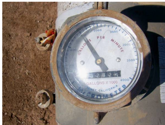
Figure 5 – Like many deep wells pumping from the Eastern Regional aquifer, Well #23 located along U.S. Highway 60 east of the community of Aguila is a productive irrigation well pumping at over 1,500 gallons per minute.
