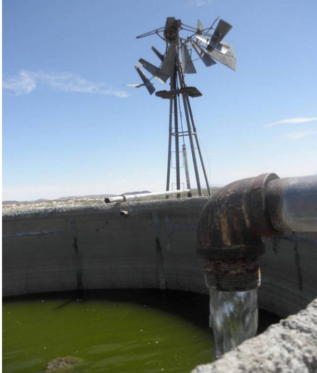
Figure 5 – Water pumped from Dun Well (RAN-52) pours into a nearby water tank formerly served by a windmill. Ranchers in the basin prefer using submersible pumps powered by portable generators to supply water for livestock.
