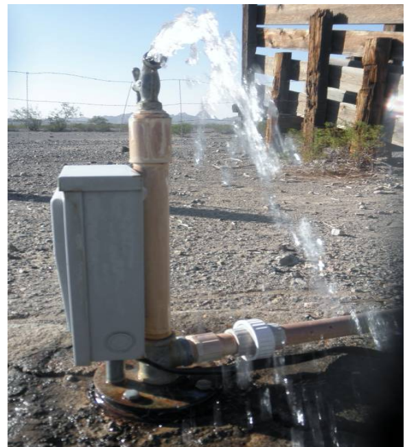
Figure 8 – The faucet on Plamosa Well (RAN-16) provides a perfect sampling location to obtain freshly pumped groundwater. The arsenic concentration at the well, 0.034 mg/L, exceeded the water quality standard of 0.010 mg/L.
