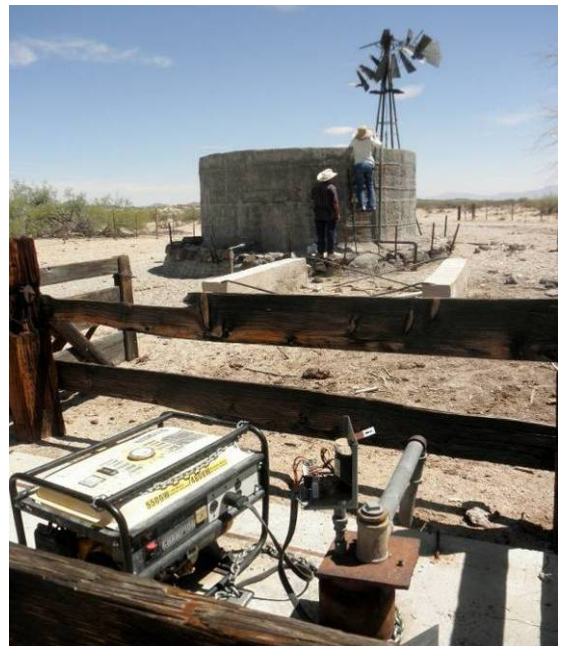
Figure 4 – Dun Well (RAN-52) is used for stock watering south of the Town of Bouse. Originally a windmill was used to fill the water tank; currently a submersible pump powered by a portable generator supplies water.
