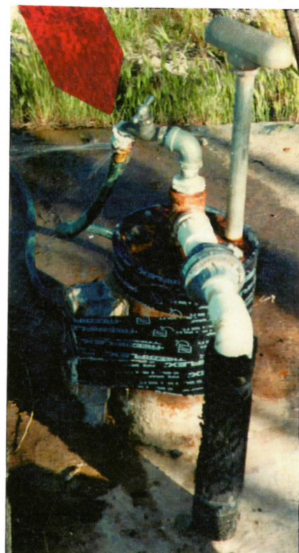
Figure 6. The red arrow points out the precipitation of calcium carbonate on a spigot as a result of very hard water pumped by a well tapping the LTL aquifer.
