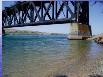
View upstream from Outfall
