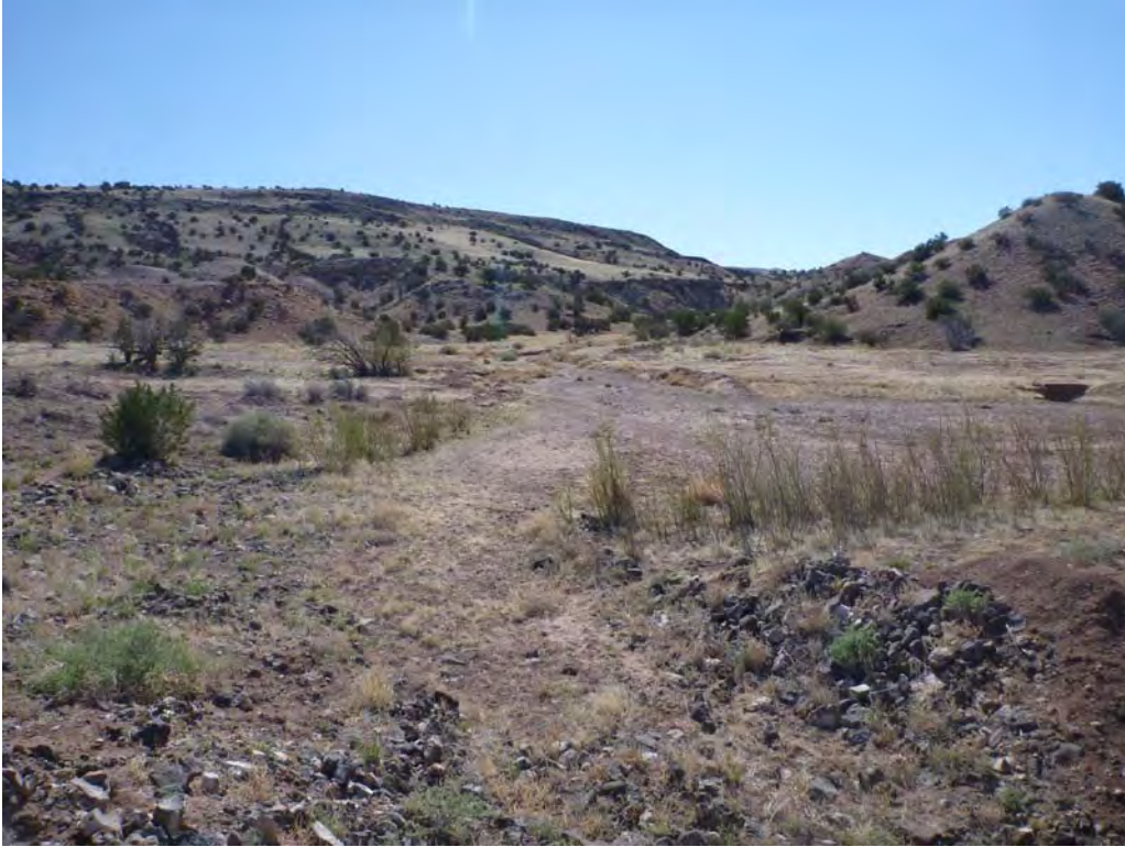
Figure 1. looking upstream across the water and sediment basin.
