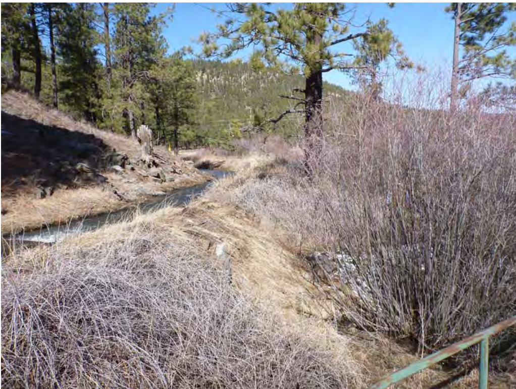
Figure 2. A portion of the hillslope that erodes when the canal freezes over and water spills out.
