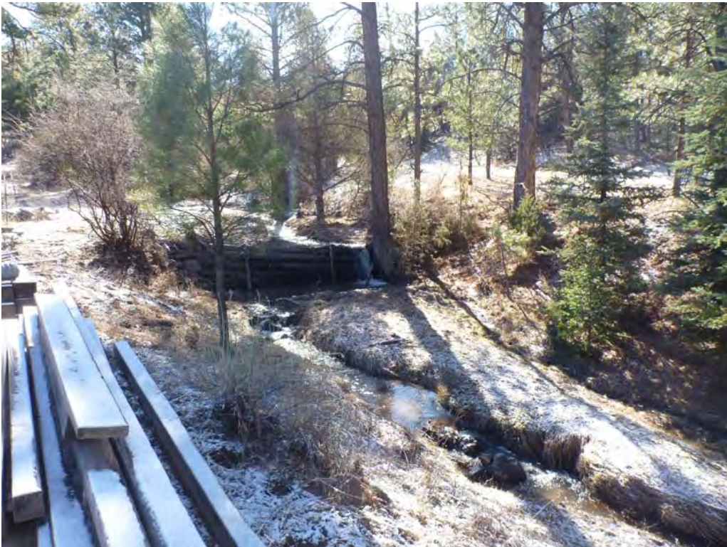
Figure 2. Temporary log structure installed to prevent further erosion of the channel.
