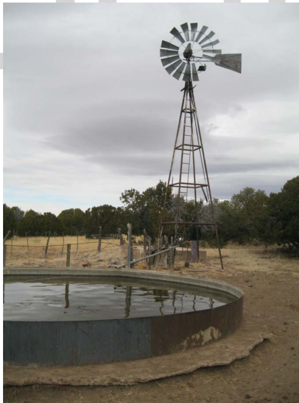
Picture of a damaged windmill and well in need of rehabilitation.
