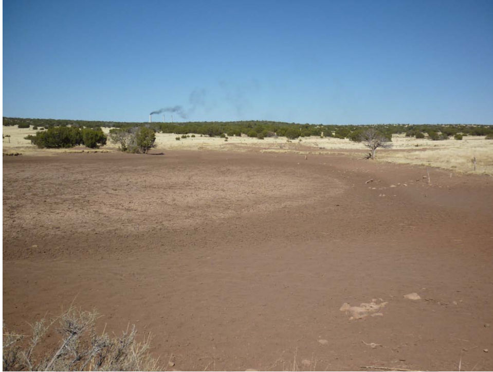
A typical sediment basin found on this ranch. This one in particular has been in service for over 20 years and is still functioning, though it needs some rehabilitation to restore its historic capacity.
