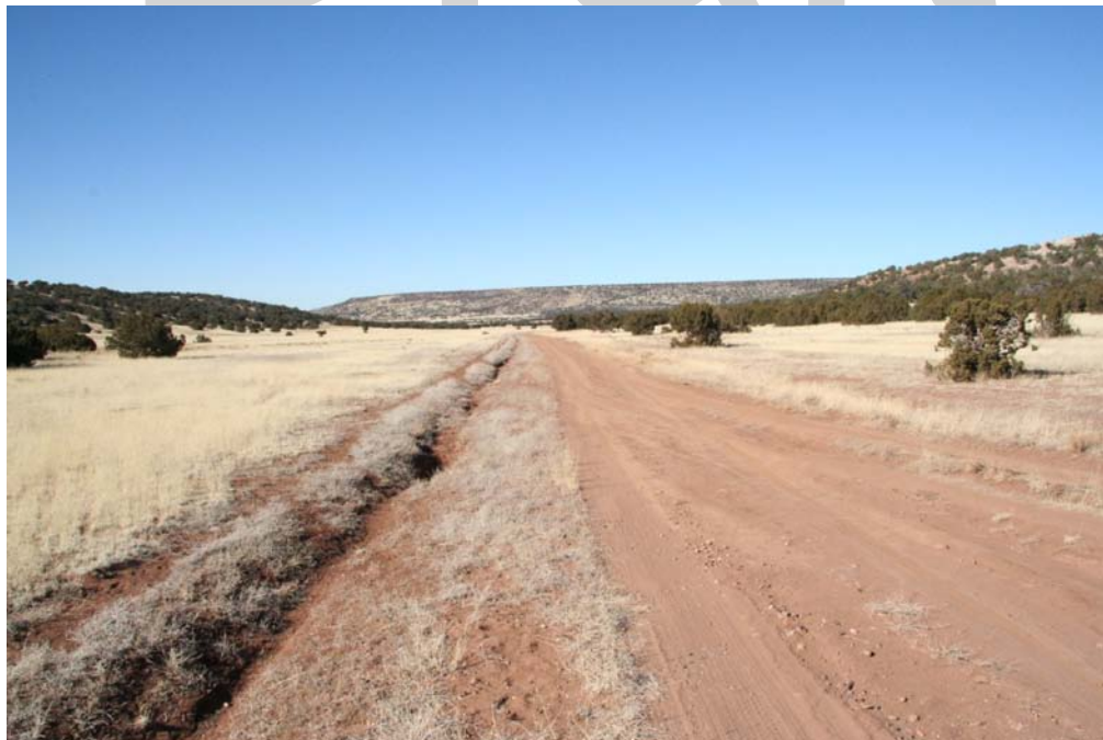
A typical road on this ranch with an actively eroding parallel gully.
