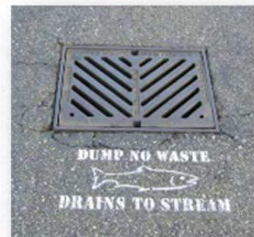
Above: An example of a storm drain stencil
