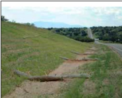
Bank Stabilization and Erosion Control along a highway
