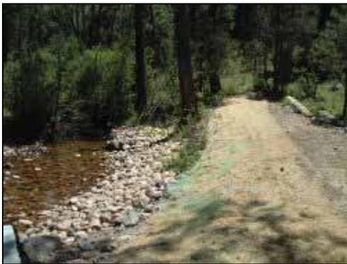
Rock Riprap and Jute Matting Erosion Control along a stream.
