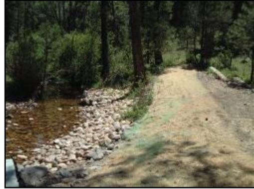
Figure 3-6: Rock Riprap and Jute Matting Erosion Control along a stream.
