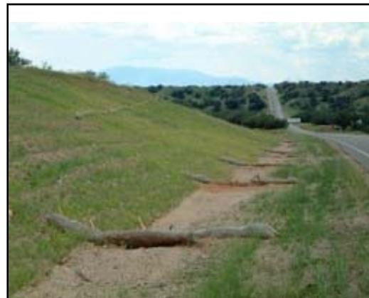
Figure 3-7: Bank Stabilization and Erosion Control along a highway
