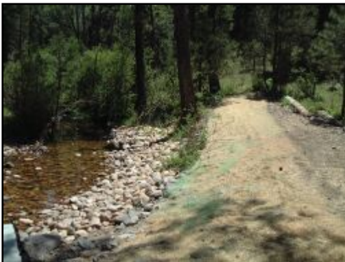
Figure 3-6: Rock Riprap and Jute Matting Erosion Control along a stream.
