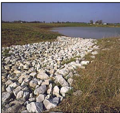
Figure 3-2: Rock Rip-Rap Sediment Control (Dept. of the Interior, Office of Surface Mining, http://www.osmre.gov/ocphoto.htm )
