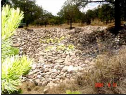
Rock riprap for erosion control (CONAFOR).
