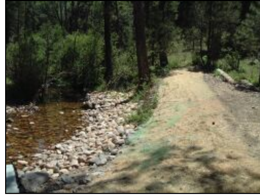
Rock Riprap and Jute Matting Erosion Control along a stream. (Photo: Lainie Levick)
