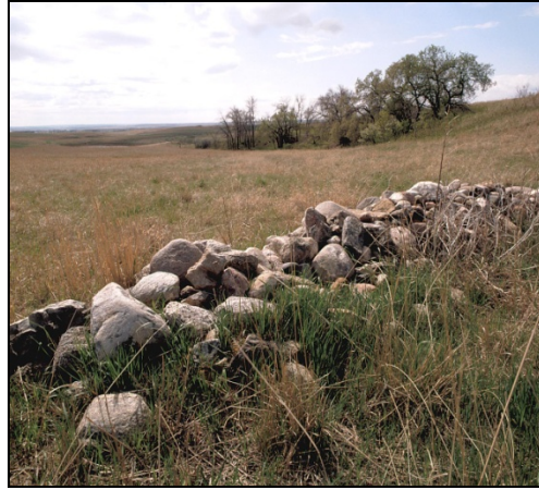
Rock Structure for Runoff Control (Dept. of the Interior, Office of Surface Mining, http://www.osmre.gov/ocphoto.htm )
