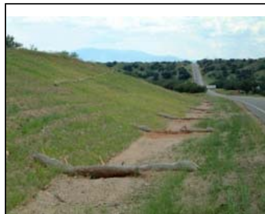
Figure 3-6: Bank Stabilization and Erosion Control along a highway
