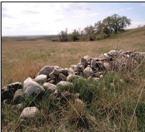
Figure 3-3: Rock Structure for Runoff Control
