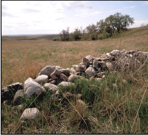
Figure 3-3: Rock Structure for Runoff Control
