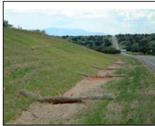
Bank Stabilization and Erosion Control along a highway (Photo: Lainie Levick)
