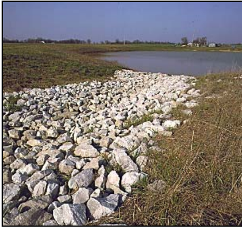
Rock Rip-Rap Sediment Control (Dept. of the Interior, Office of Surface Mining, http://www.osmre.gov/ocphoto.htm )
