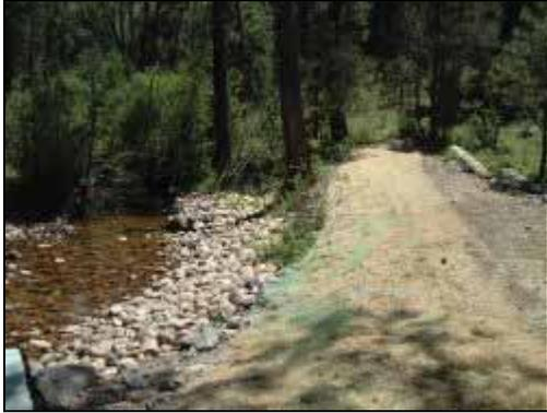
Rock Riprap and Jute Matting Erosion Control along a stream.
