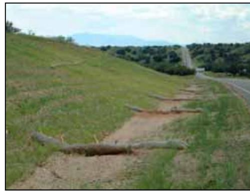
Bank Stabilization and Erosion Control along a highway
