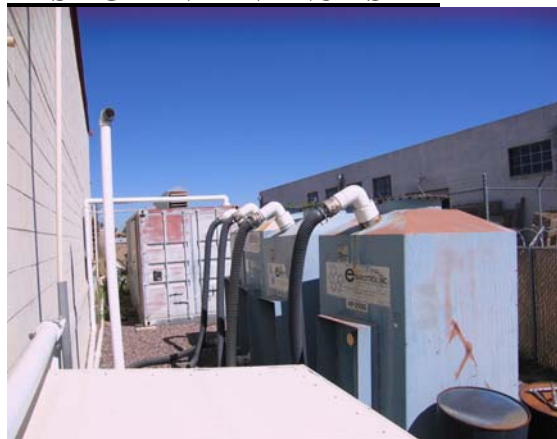
Soil Vapor Extraction System at VW&R Facility
