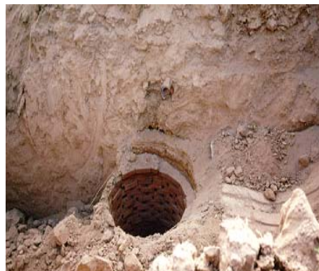
Seepage Pit that was removed from the West Osborn Complex Site
