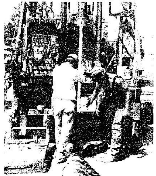
Drilling of a monitor well in the West Central Phoenix area. Monitor wells are installed to determine such things as the direction in which groundwater flows and the types and amounts of contaminants present.
