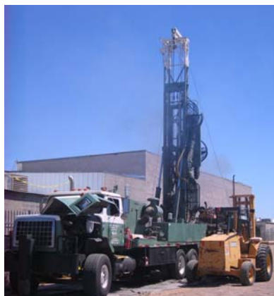
Placement of new monitoring well North Plume site
