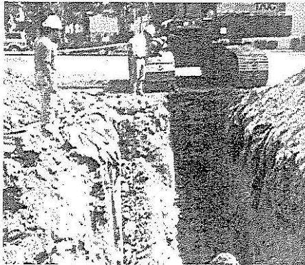
This photograph shows a seepage pit found during the trenching activities at the West Osborn Complex.
