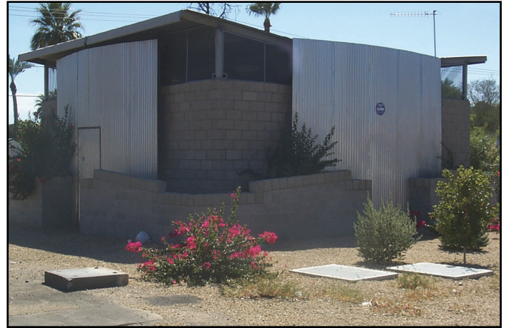
Central and Camelback Groundwater Treatment Plant.
