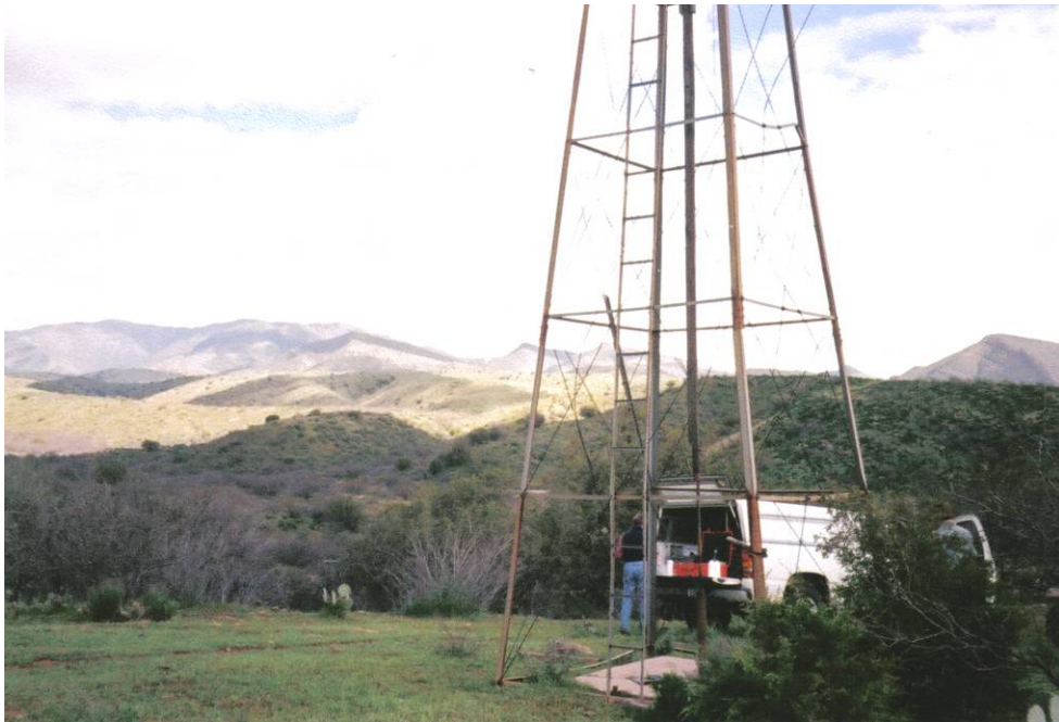
Figure 9 – A 392-foot-deep Challenger windmill (DSW-9) provides water for domestic and stock uses in an upgradient area of the basin. The sample from the well contained hard water but met all health and aesthetics based water quality standards.
