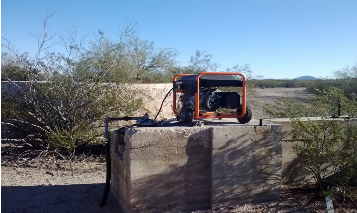
Figure 3 – A generator powers the submersible pump in Mine Pump well. Water from the well is piped to a nearby water tank and distributed to troughs for livestock and wildlife use. A split sample (TIG-1/2) was collected from the well.
