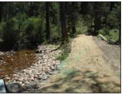
Rock Riprap and Jute Matting Erosion Control along a stream. (Photo: Lainie Levick)
