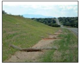
Figure 3-7: Bank Stabilization and Erosion Control along a highway (Photo: Lainie Levick)
