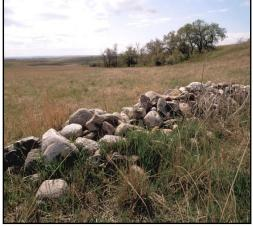
Figure 3-3: Rock Structure for Runoff Control (Dept. of the Interior, Office of Surface Mining, http://www.osmre.gov/ocphoto.htm)
