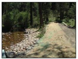
Figure 3-6: Rock Riprap and Jute Matting Erosion Control along a stream. (Photo: Lainie Levick)
