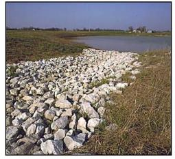
Figure 3-2: Rock Rip-Rap Sediment Control (Dept. of the Interior, Office of Surface Mining, http://www.osmre.gov/ocphoto.htm)
