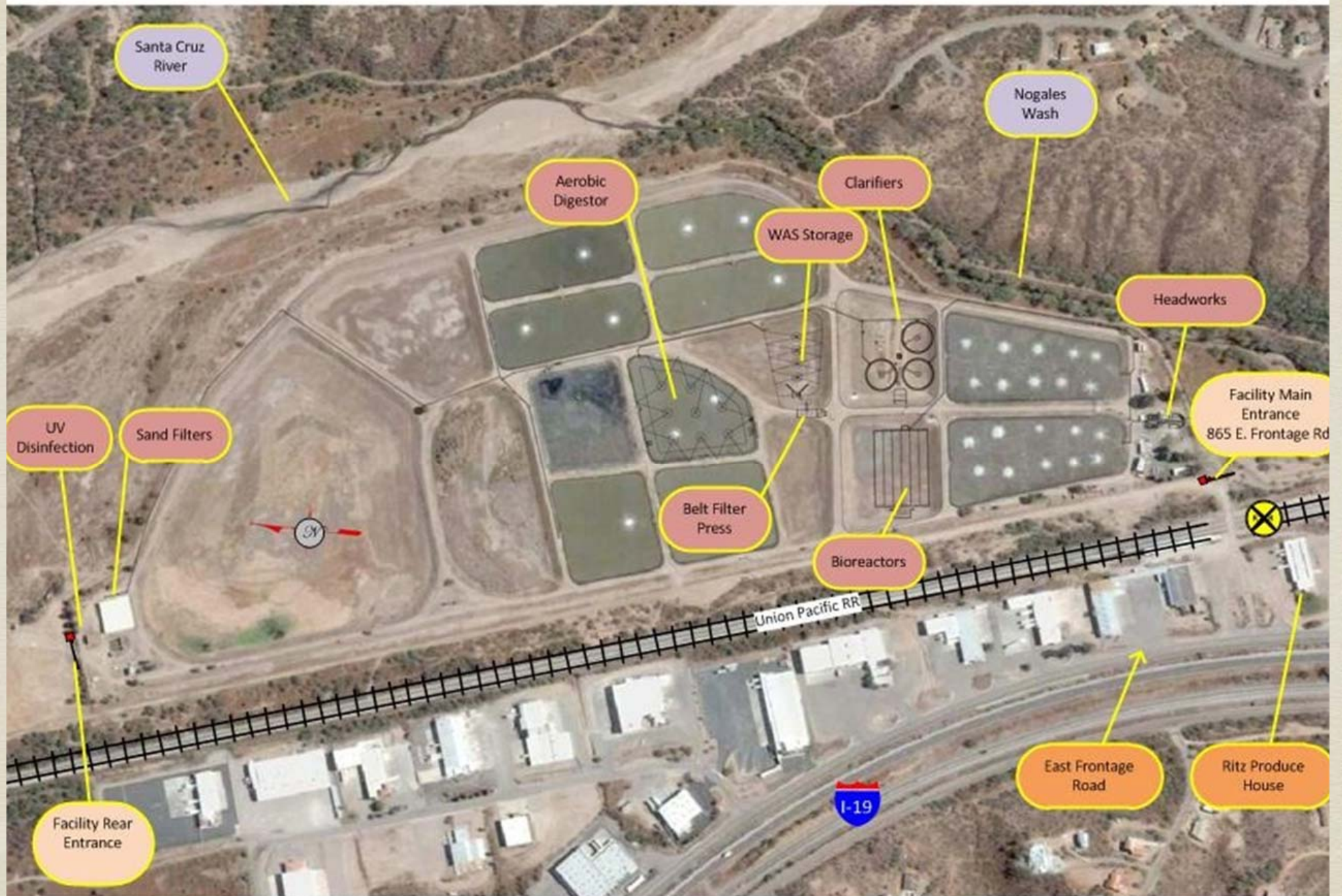
Nogales International Wastewater Treatment Plant (NIWTP) 865 East Frontage Rd., Rio Rico AZ 85648
